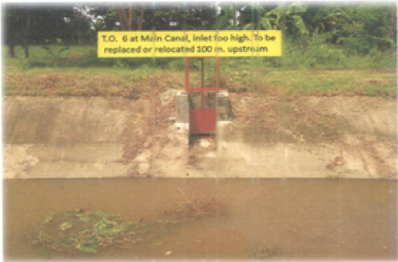
Figure 4- 3 Wrongly located and positioned turnouts in Banaoang PIS, a common faulty design outcome that results in corresponding O&M problems in irrigation system
