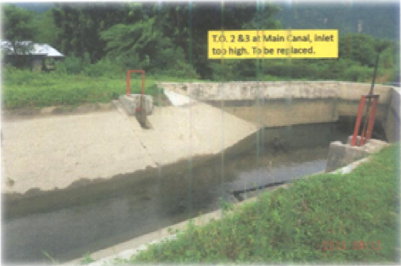
Figure 4- 3 Wrongly located and positioned turnouts in Banaoang PIS, a common faulty design outcome that results in corresponding O&M problems in irrigation system
